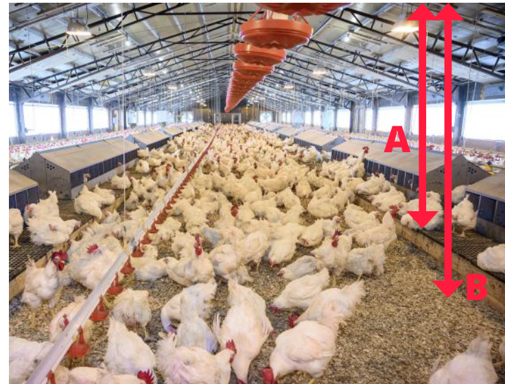
Airspeed uniformity is also affected by the height differential between the drop ceiling or roof and the scratch and slat areas. Prevent large differences in height between slat and the ceiling (A) compared with the scratch area and the ceiling (B).
