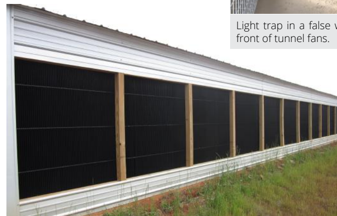
Tunnel inlet light trap.
